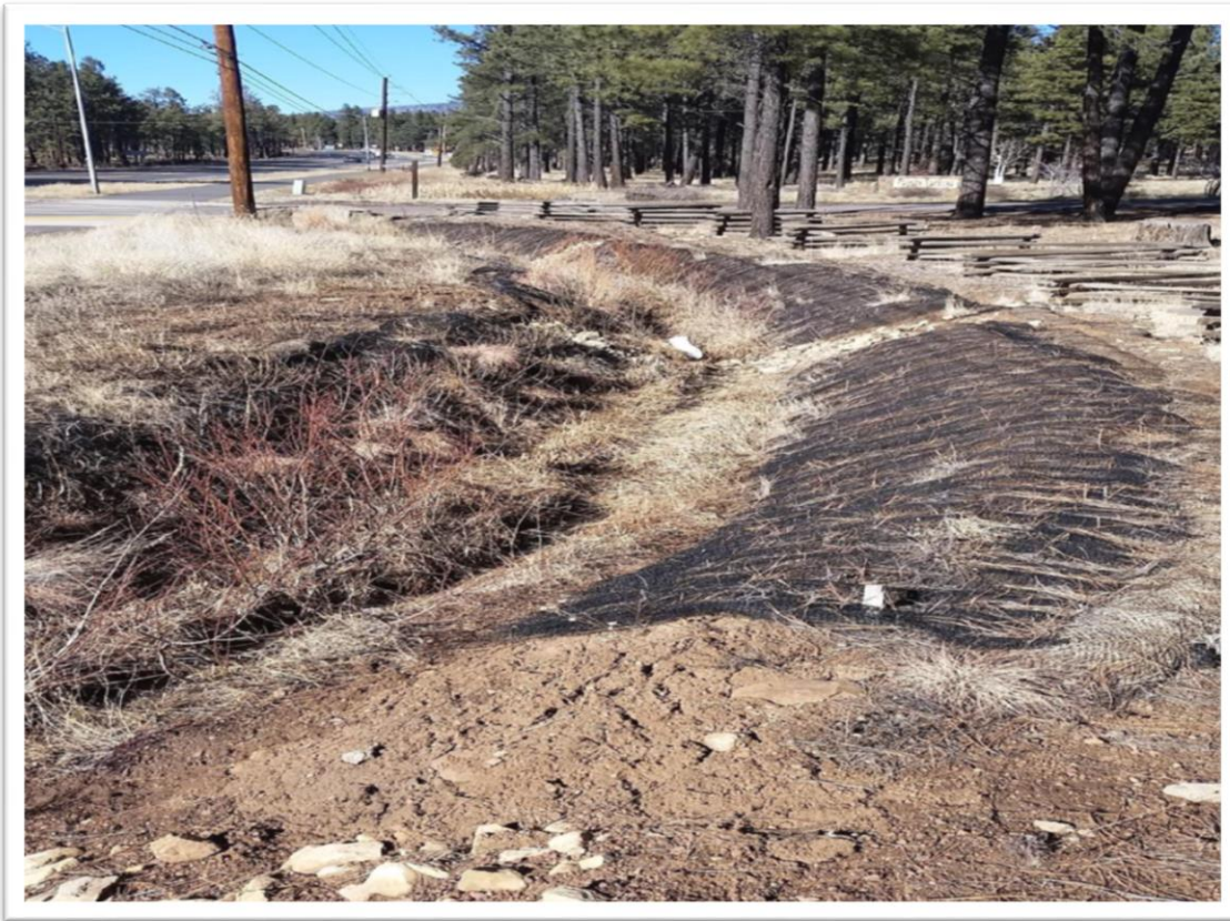
Figure 4: Turf reinforcement matting on downstream end of stream
